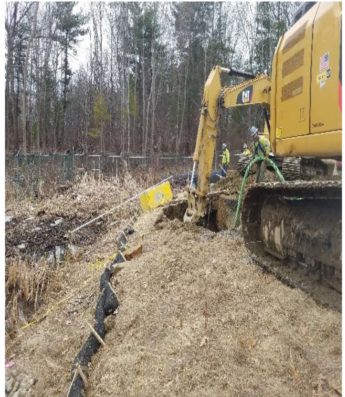
Fig 24: Crew beginning to excavate for Str. 125 foundation. Viewing west. (02-26-20).
