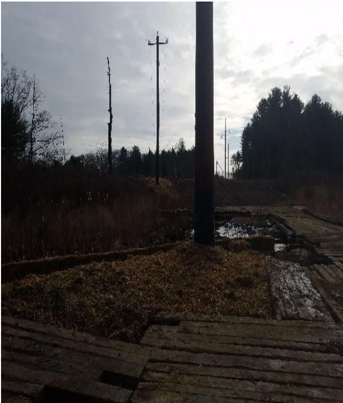
Fig 23: Str. 114 foundation. Viewing east. (02-26-20).
