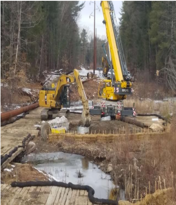
Fig 19: Str. 114 work area. Viewing west. (02-25-20).
