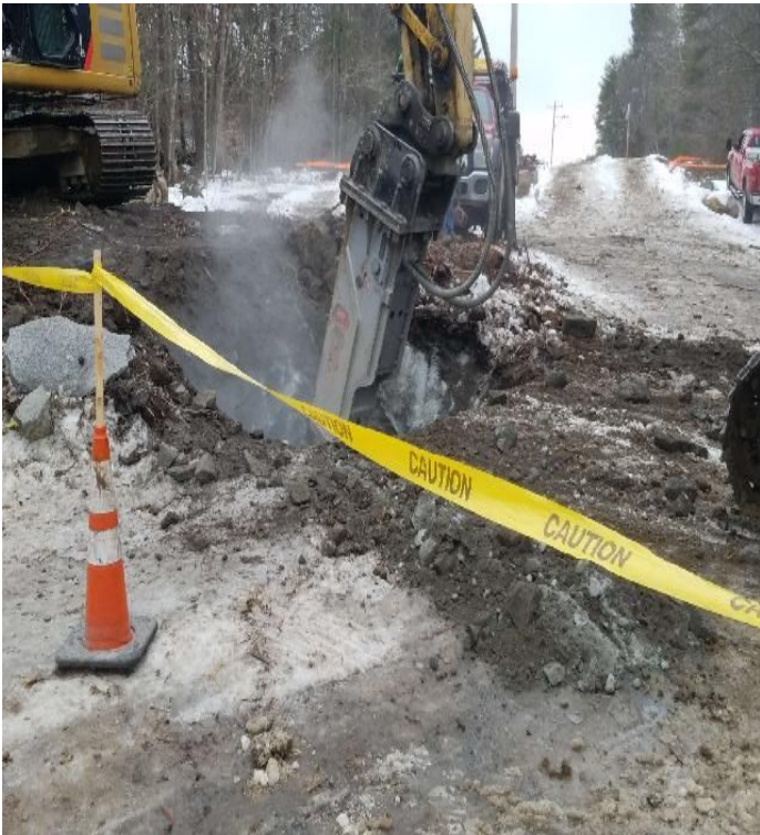
Fig 15: Hammering ledge at Str. 66. Viewing west. (02-25-20).
