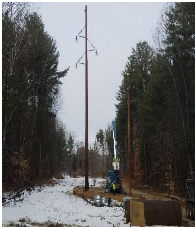
Fig 20: Str. 113. Viewing west. (02-25-20).
