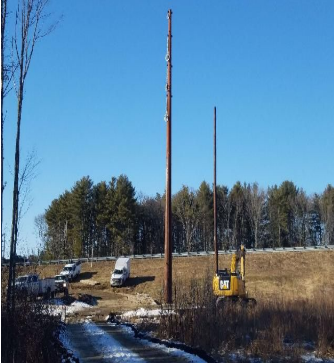
Fig 9: Str. 117. Viewing west. (02-21-20).
