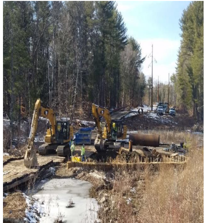
Fig 14: Crew beginning to excavate foundation for Str. 114. Viewing west. (02-24-20).
