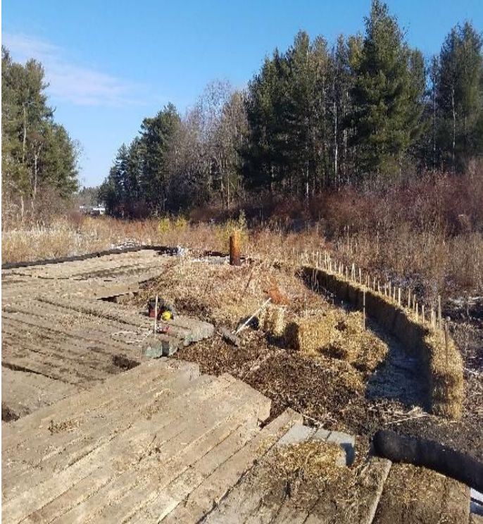
Fig 13: Str. 114 work area. Viewing north. (02-24-20).
