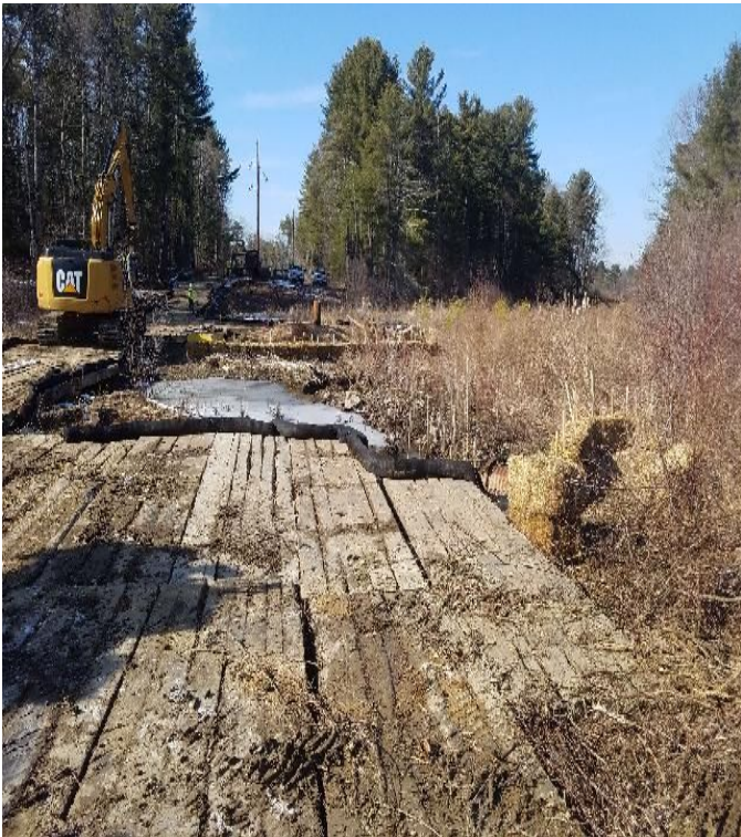
Fig 11: BMPs below Str. 3850-64 location. Viewing west. (02-24-20).
