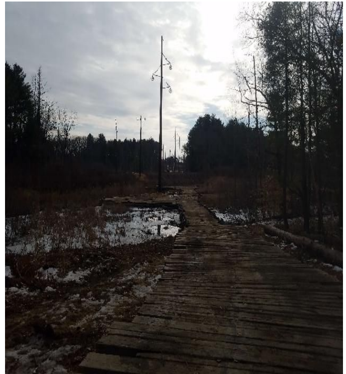
Fig 22: Access road to Str. 114. Viewing east. (02-26-20).
