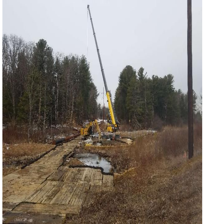
Fig 18: Prepping to raise Str. 114. Viewing west. (02-25-20).
