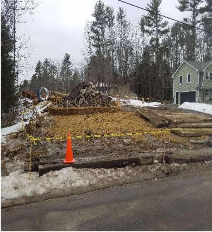
Fig 21: BMPs installed around rock pile at Str. 67. Viewing west. (02-25-20).
