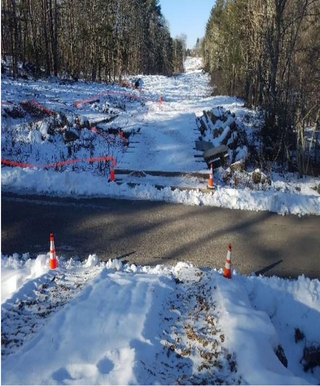
Fig 5: Access road crossing over Timber Brook Lane. Viewing west. (02-21-20).
