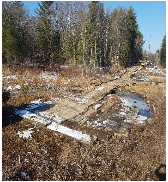
Fig 10: Access road to Strs. 114 and 3850-64, through wetlands NW17 & NW51N. Viewing west. (02-24-20).
