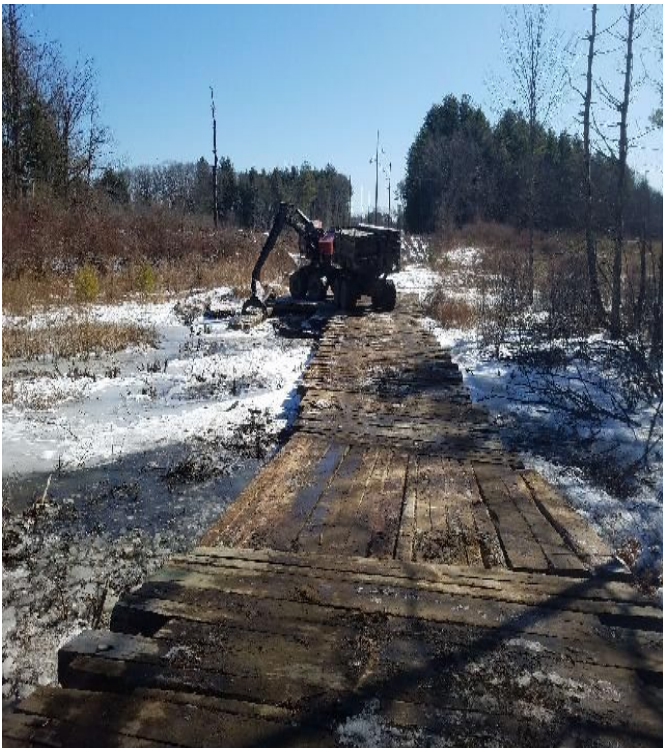
Fig 7: Building access road through wetland NW17 and NW51N. Viewing east. (02-21-20).
