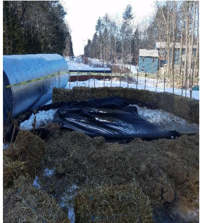
Fig 2: Dewatering basin set up at Str. 67. Viewing west. (02-20-20).
